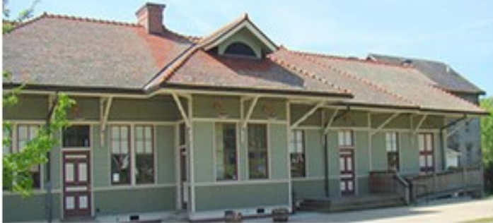
Restoration of the Historic L and N Railroad Depot circa-1910, Depot Street, Stanford, Kentucky
