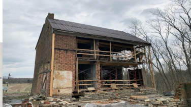
Newland east wall restored with Whitley House diamond pattern brick work and stone foundation.
