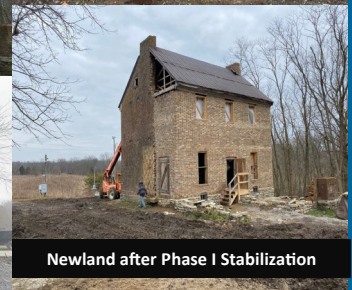
Newland east wall restored with Whitley House diamond pattern brick work and stone foundation.
