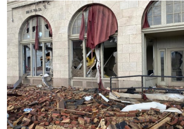
Riley Architect Services' Office After the Tornado.
